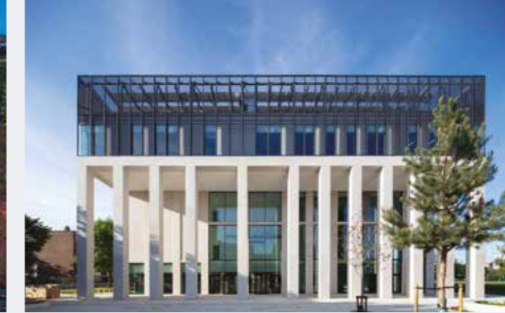
Britannia Leisure Centre, Secondary School and Sixth Form, City of London Academy, Hackney
