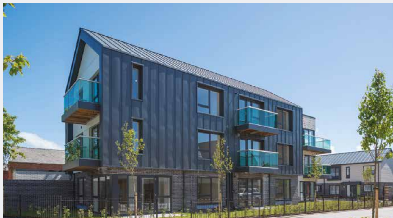
North West & North Wales Region, Queens Park, Blackpool
