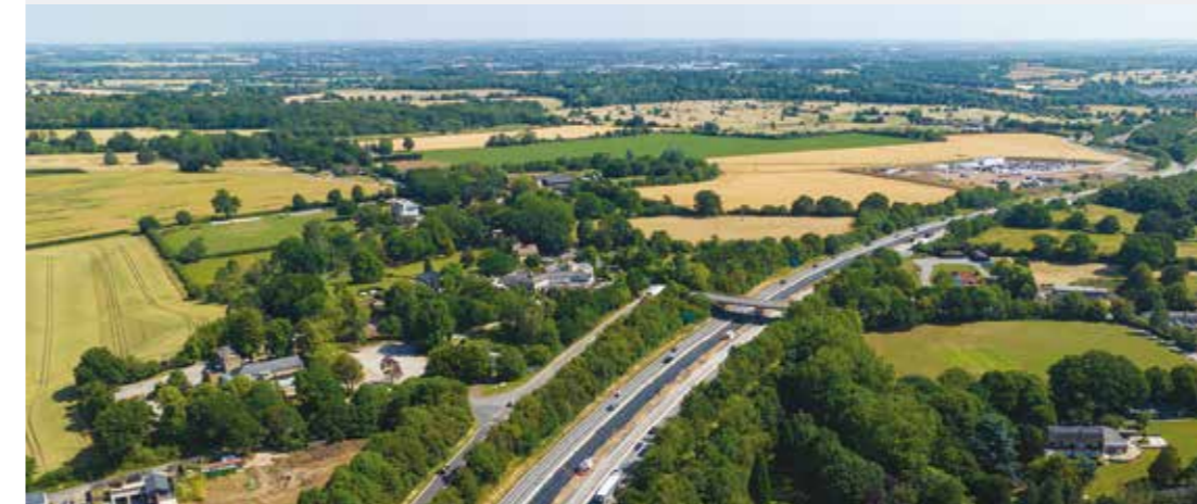
A12, Essex Reconstruction Works
