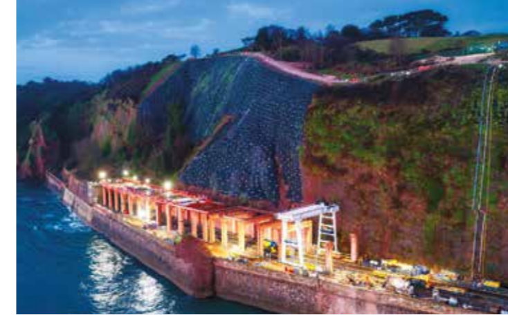
Parsons Tunnel Upgrade under South West Rail Resilience Programme
